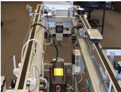
Each conveyor section is equipped with its own controller and motor drive.
